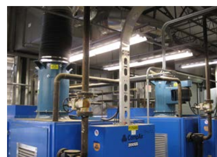
Air Compressor Heat Exhaust Fans
