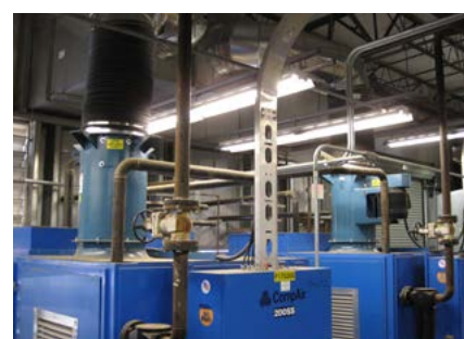
Air Compressor Heat Exhaust Fans
