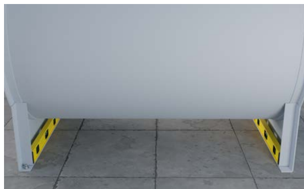
Carefully level the fan on the foundation
