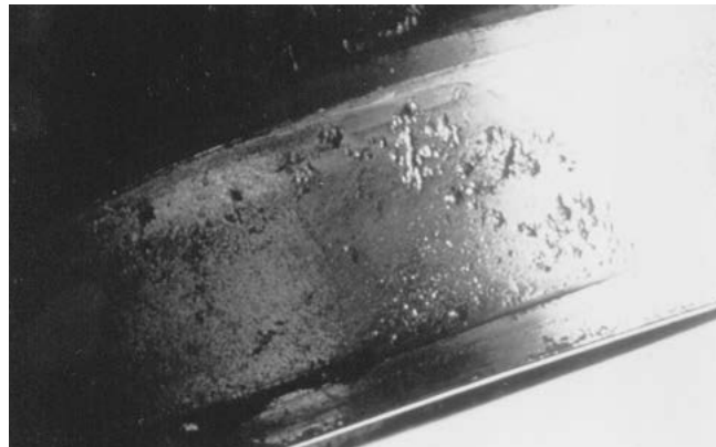
Figure 7. Spalls & Wear Patterns in the Race
