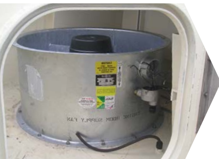
Engine Room Supply Fan (Marine)
