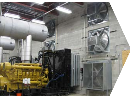
Generator Room Exhaust
