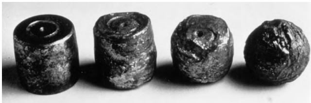
Figure 9. Damaged Spherical Bearing Rollers
